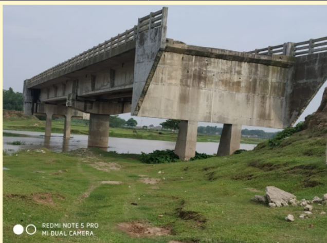
Galgalia to Pintola in Kishanganj district (Chainage 123.30)
